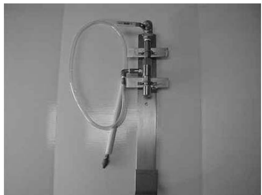
Figure 11-4 Scheme of a wall-mounted foam and rinse station that can provide foam application at convenient locations in a food plant through automatic metering and mixing of the cleaning compound. Courtesy of Ecolab, Inc., St. Paul, Minnesota.
