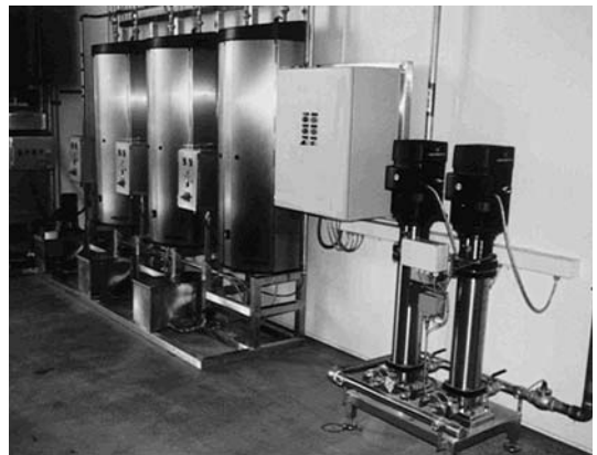
Figure 11–2 A centralized medium pressure, (boosted pressure) system for a large cleaning operation. Courtesy of JohnsonDiversey, Inc., Detroit, Michigan.
